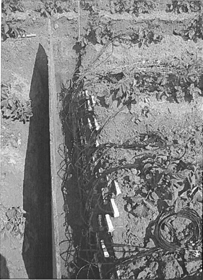
Figure 5. Plywood installed and backfill commenced.
